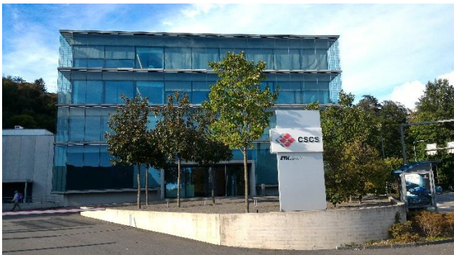
Photo 3 Swiss supercomputer center (CSCS)
